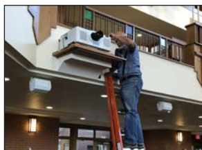
Installing New Projectors
